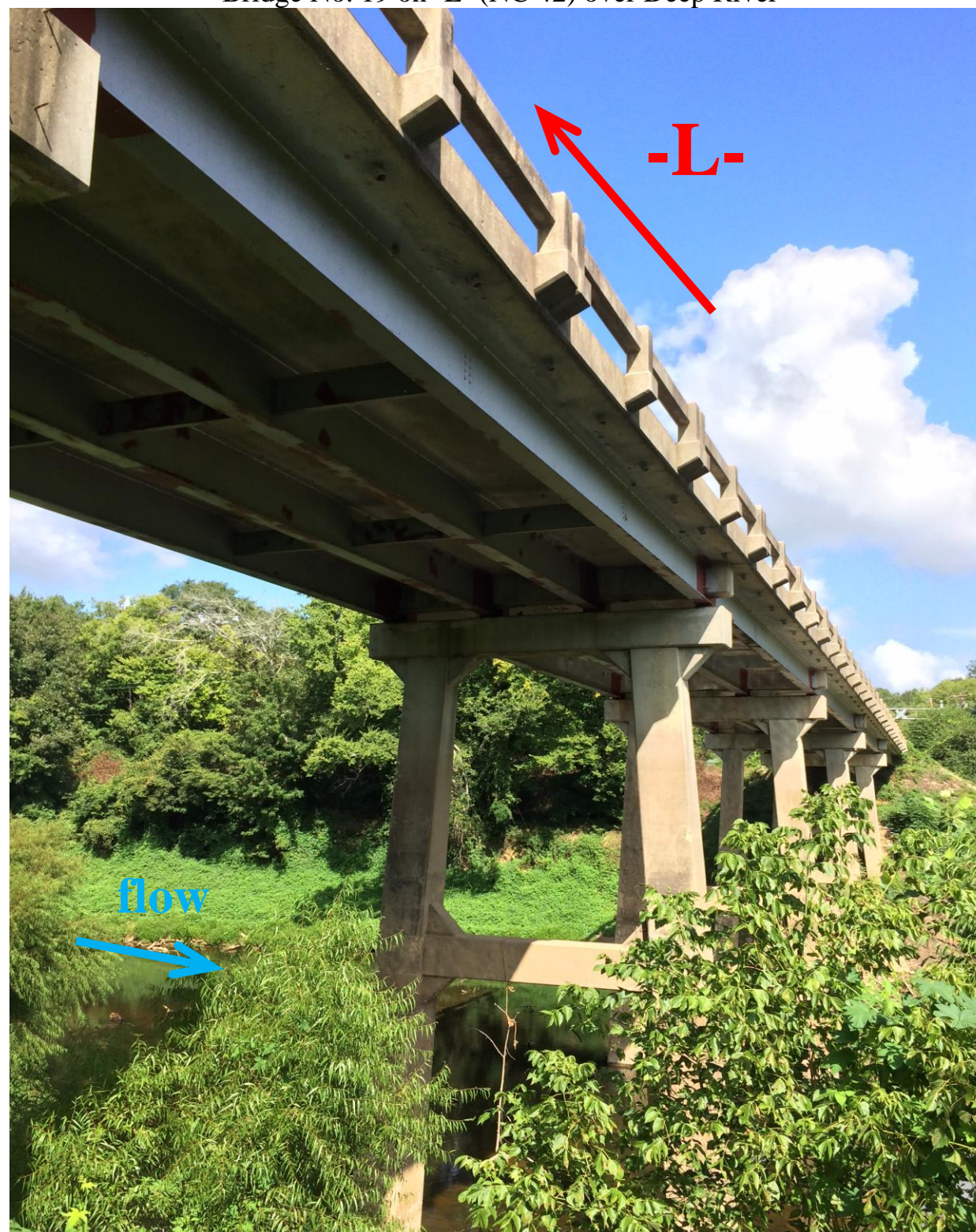
Looking Northwest towards End Bent 1
